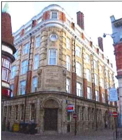
City Buildings, Fish Street
